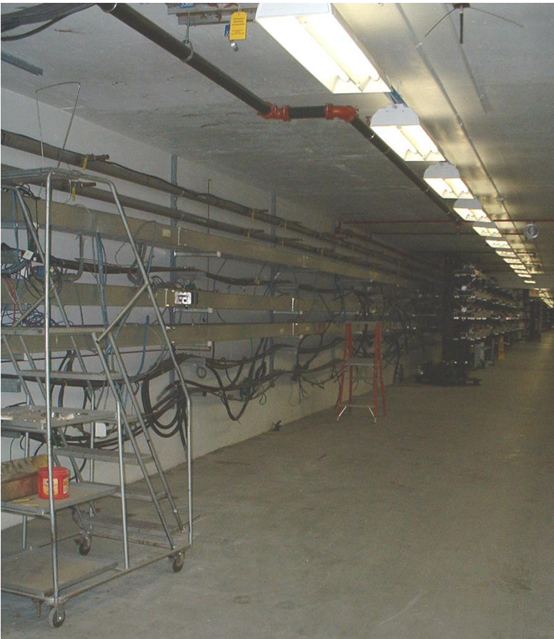
West Spreader Removal
