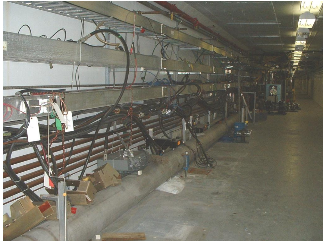
West Recombiner/OR Removal
